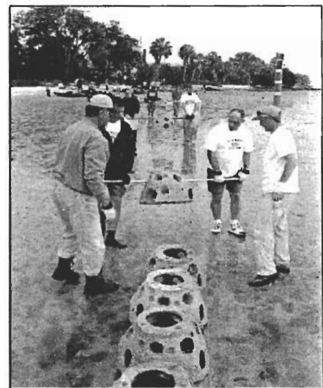
Installation of Oyster Domes for Phase I at MacDill
