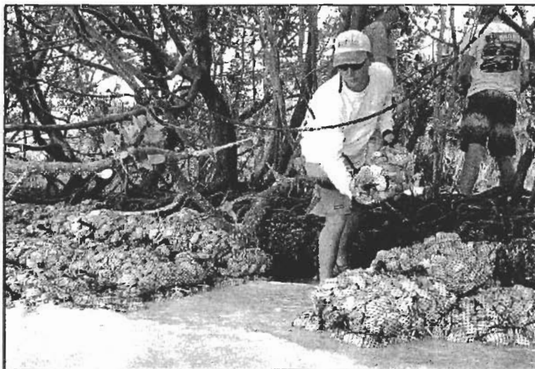
Phase II included bolstering the eroding stand of black mangroves with oyster shell bags.
