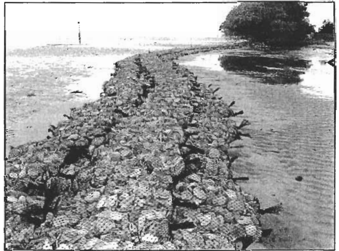
150' oyster shell bar installed during Phase II
