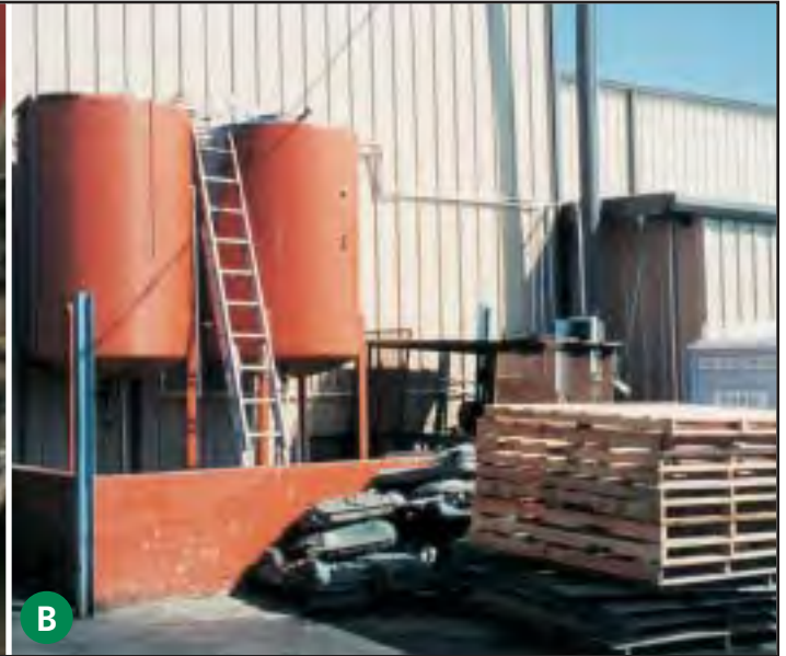
A – Wash table for engine parts over an impervious surface draining to an oil-water separator; B – Wastewater capture, recycle and reuse storage system inside secondary containment.
