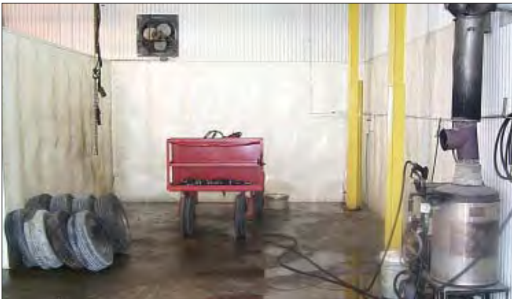
An enclosed pressure washing area, over concrete, with wash water drained through an oil/water separator.
