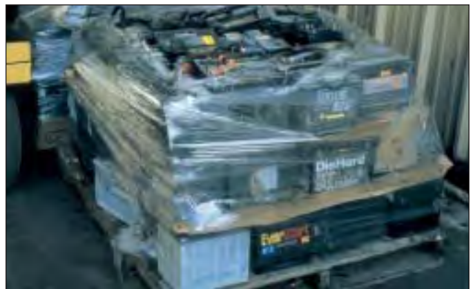
Plastic wrapped lead acid batteries piled less than 4-high on a pallet, on an indoor impervious surface, notice the use of cardboard between layers of batteries.
